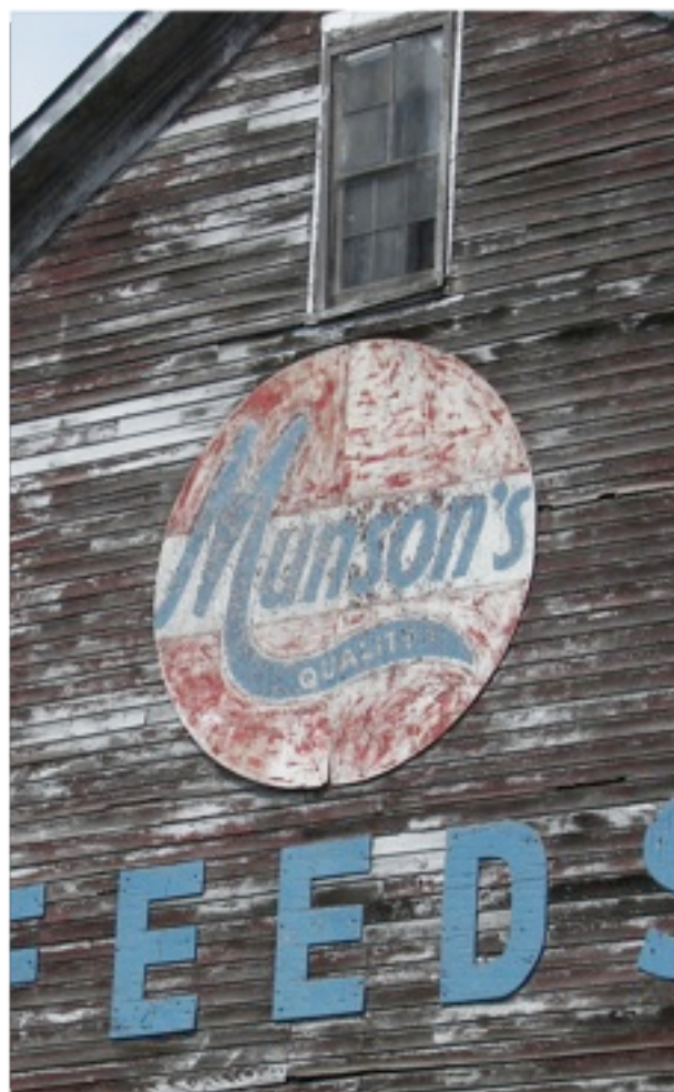
WCHS Staff documented the demolition of the Munson Feeds Elevator July 29 & 30. Look for more pictures and information online and in our next newsletter.
